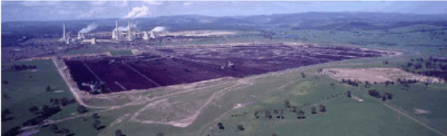
Figure 1(a): Surface Brown Coal Mine and Electricity Generation Units
