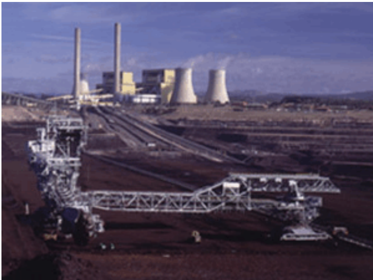
Figure 1(b): Mining Shovel and Transport Facility
